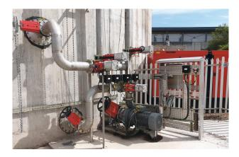
In the first stage of the mixing process, the liquid will be injected into the upper half of the tank, while biogas is aspirated from the top of the tank and mixed into the liquid.
