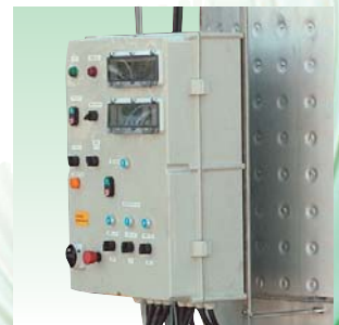
PLC-controls, regulates, monitors and registers
