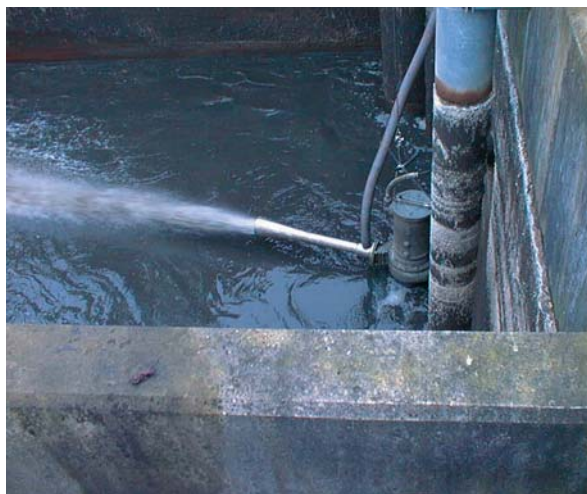
Storm water tank cleaning
