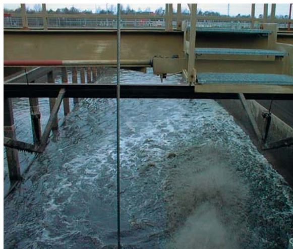
Storm water tank cleaning
